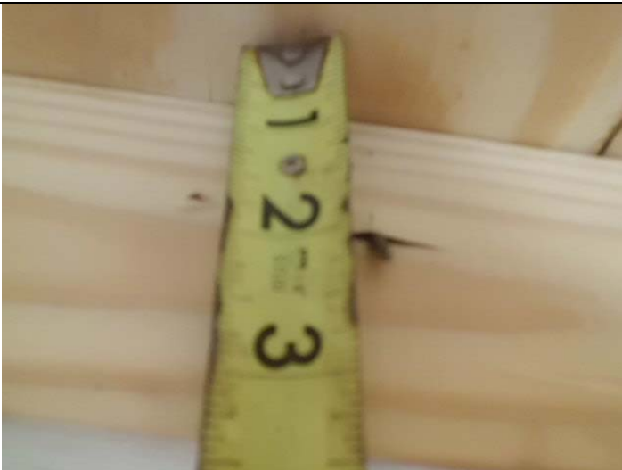
Roof deck attachment
