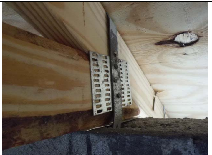
Roof to wall attachment
