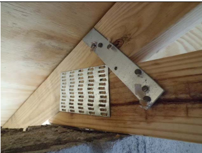
Roof to wall attachment
